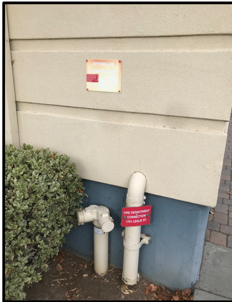
Exterior and interior sprinkler controls
